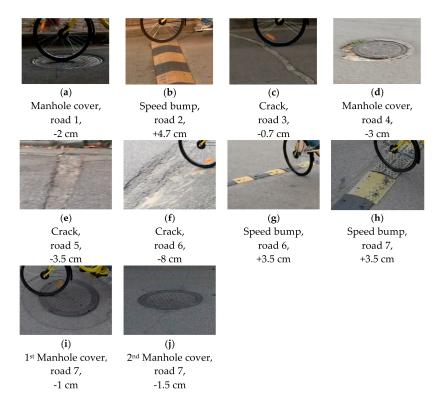
Figure 11. Potholes and humps on the seven road sections, as well as their types and longitudinal offsets.
